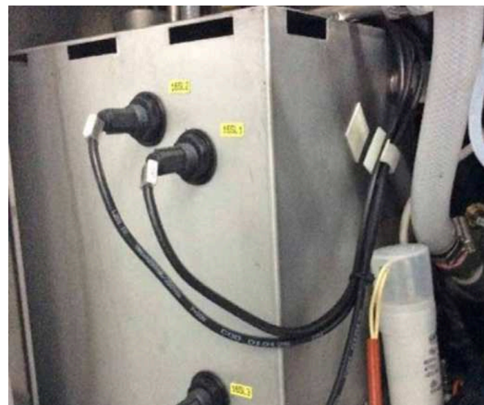
Figure 1b. Break-tank and associated pipes
